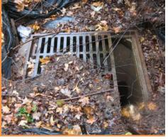
Figure 4.3-1 Missing Proper Cover
