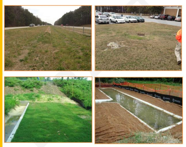
Figure 5.1-1 Channel between Filter Strip (top left), Filter Strip around Drop Outlet (top right), Concrete Level Spreader and Filter Strip (bottom left), and Concrete Level Spreader under Construction (bottom right)
