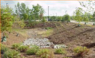
Figure 5.6-1 Dry Detention Basin with Low-Flow Channel (left) and Dry Detention Basin with Landscaping (right)
